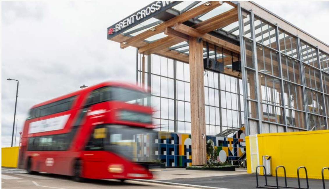
↑ Brent Cross West railway station entrance, constructed in timber.
